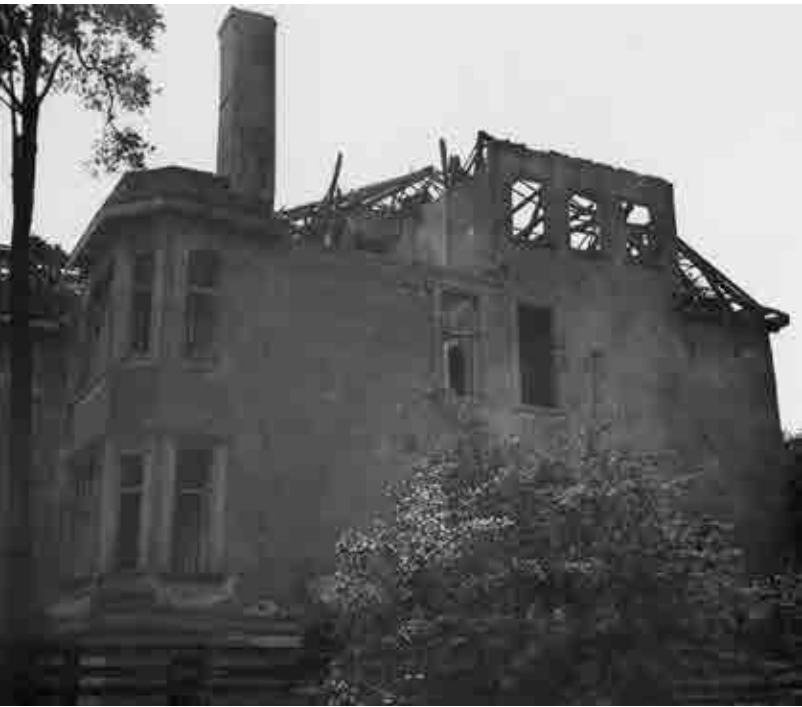
Fig. 1.33 Bombed-out Building Lassenstraße 26, View from the Garden / Ruine Lassenstraße 26, Gartensicht Photo not dated / Foto undatiert Landesarchiv Berlin B Rep 209-01 94-13746
